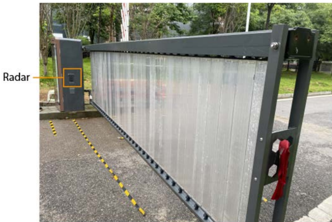
Figure 3-4 Radar installation completed
